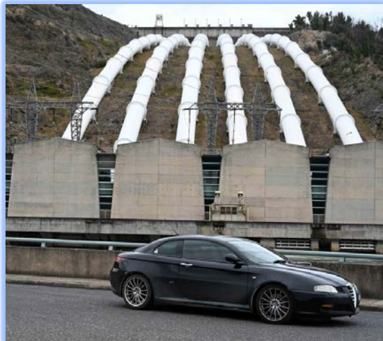
The hydro tunnel at Tumut #3 Power Station near Talbingo.
